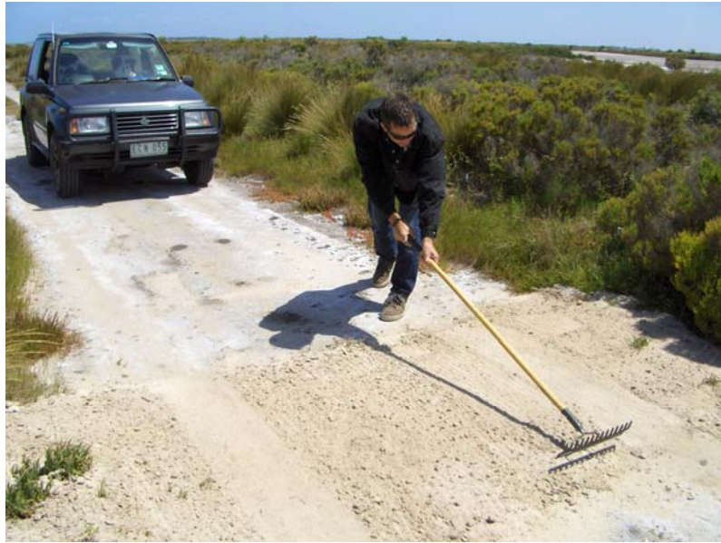
Figure 1. Installing sand pads at the Cheetham Wetlands.
